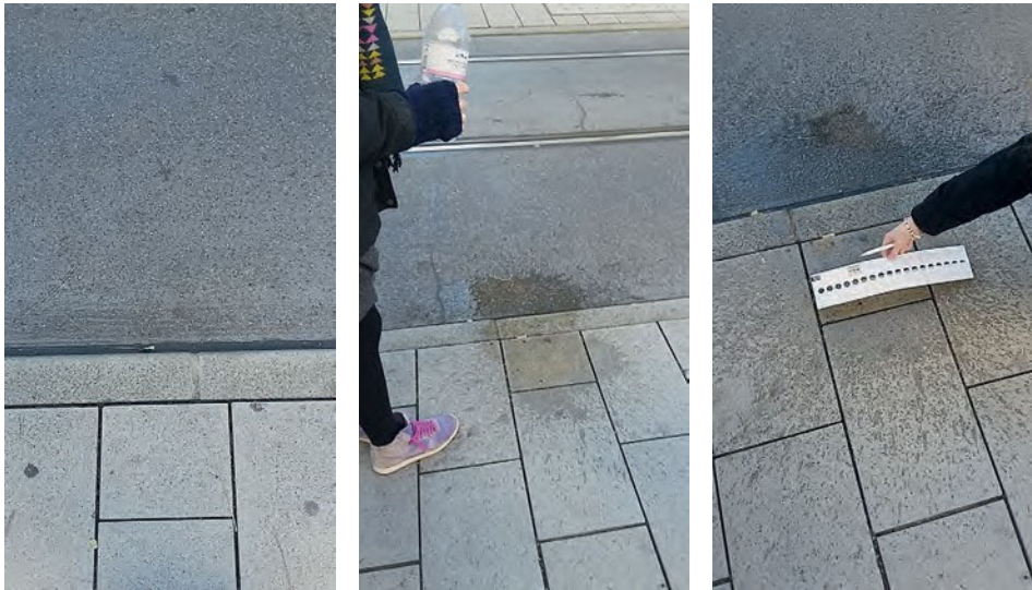
Figures 9–11 BBSB’s architect stages a demonstration of the inaccessible choice of materials and the problem it poses to identify street zoning contrasts. Left: Detail of different pavement’s (lane and sidewalk) junctions, showing different degrees of grey. Centre: A water puddle forms at the junction of both pavements after a student drops water from a flask. Right: The BBSB architect uses the lightness meter grid to measure the contrast of all wet pavements
