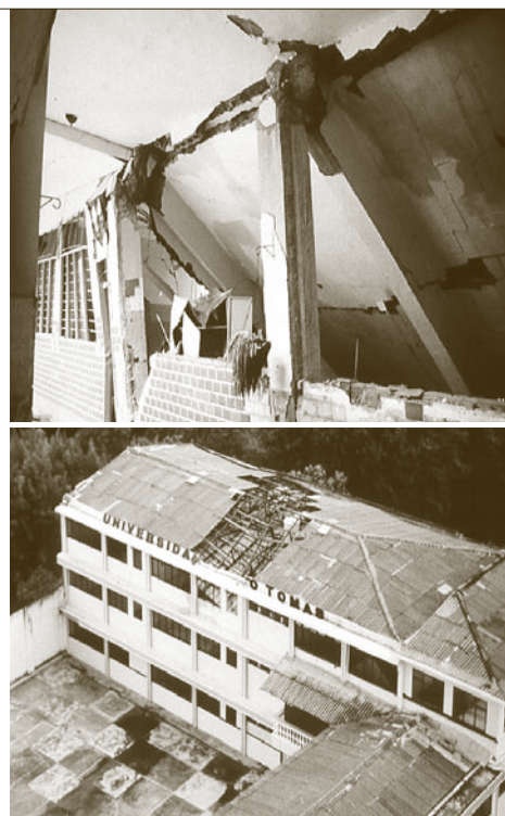
Figure 1 Building damage in educational facilities after the 1999 Quindío earthquake in Colombia
