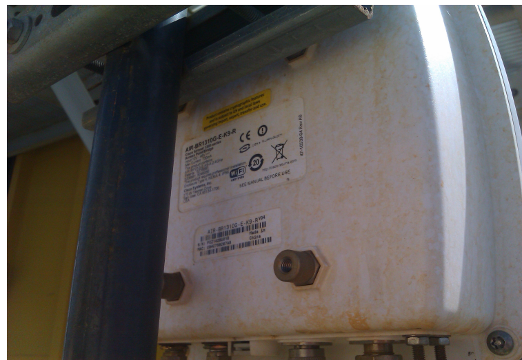
Illustration 8. Photos of one end of a wireless point to point link
