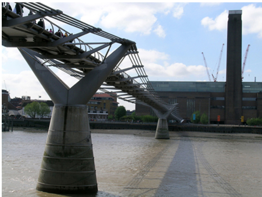
Figura 8. Bill Fontana (2006). Harmonic Bridge .
