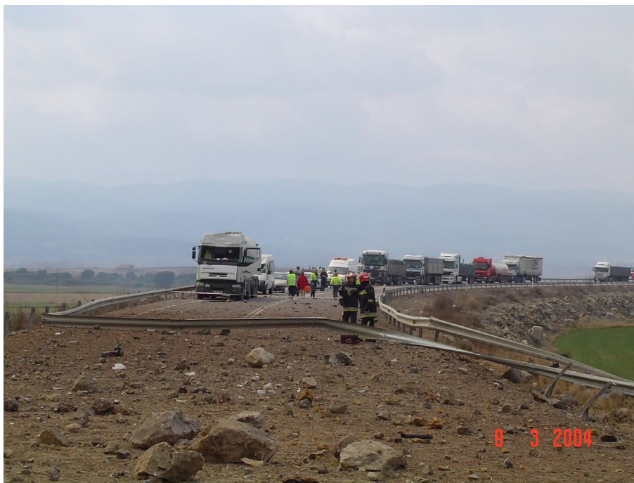
FIGURE 2 Crater caused and guardrails blown off by the explosion 50
