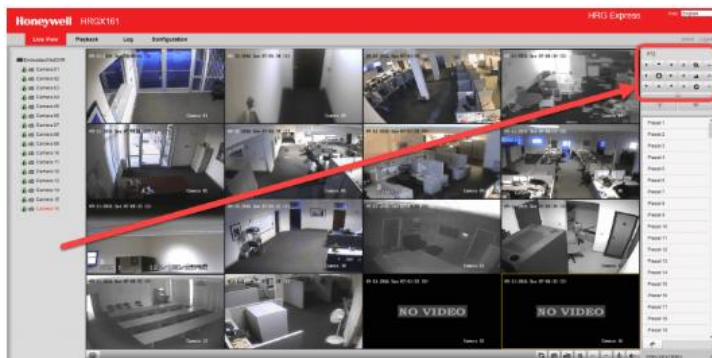
Figura 17 – Panel de control de Honeywell
